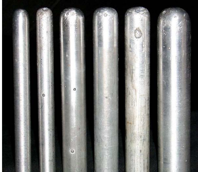
Figure 11 - Slight melting seen on lightning rods struck by a direct hit of lightning (Figure courtesy of R. Sonnenfeld)
