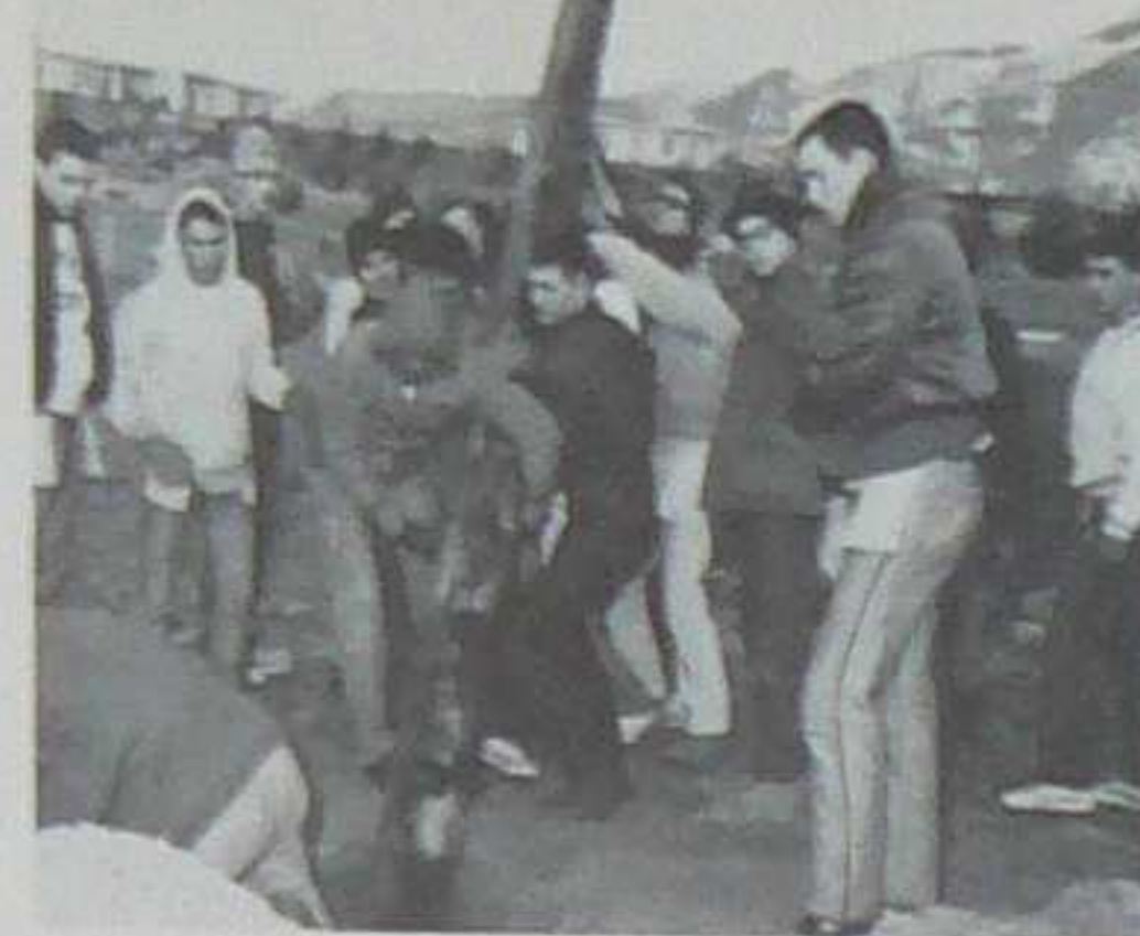
With the pole in place the green can now be hoisted (with a helping hand).
